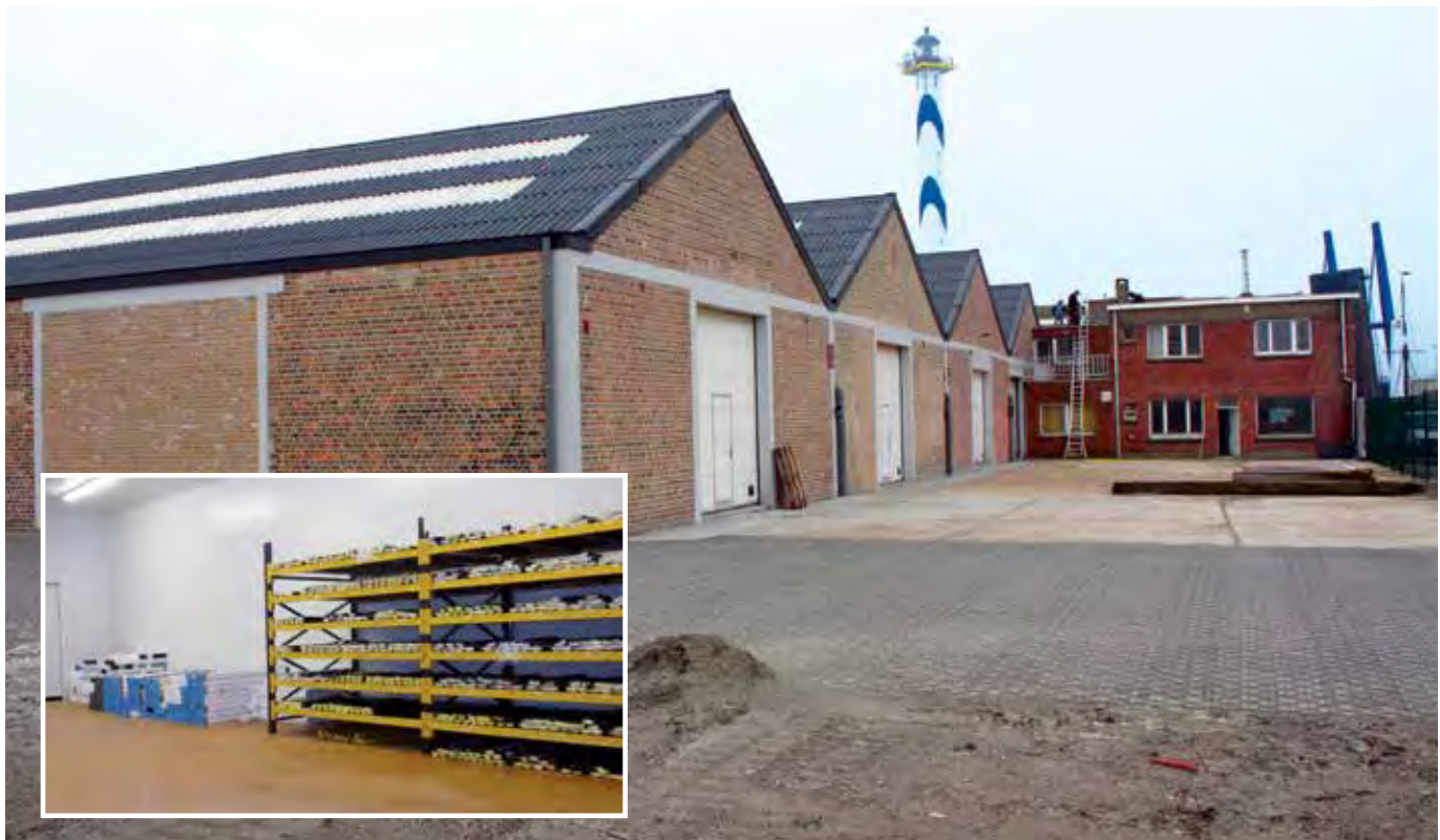
VLIZ RENOVATED THE OSTEND MARINE STATION'S FOUR WAREHOUSES AT THE HALVE MAAN SITE ON THE OSTEND EASTERN BANK. – The warehouses make it possible to develop dry and wet laboratories. The core repository (inset) was reactivated with a new cold store (measuring 12 x 6 x 3 metres) on 7 December 2012.
