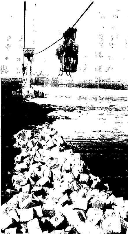
Cable railway for dike construction
