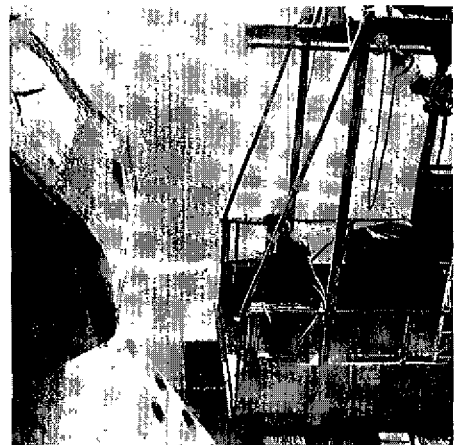
15 Protection of pier by gunnite layer
