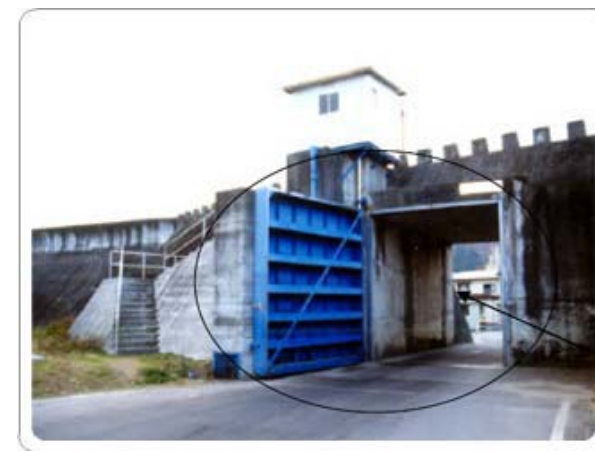
Tsunami water gate which is closed after tsunami warning is issued in Japan
