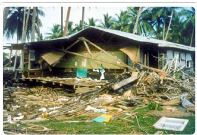
A two-story wooden school building that stood near the church at Sissano Mission was carried 65 m by the wave until caught by a grove of coconut palms. The lower floor of the building collapsed, but the upper floor class rooms were preserved. Schoolwork was still hanging on the wall. (Photo credit: Hugh Davies, University of PNG.)
