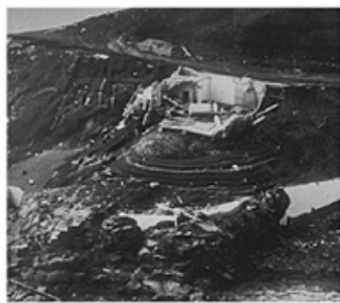
Scotch Cap lighthouse, Unimak, Alaska, before and after a 35-m high tsunami destroyed the 5-story lighthouse on 1 April 1946. The tsunami also caused death and damage in Hawaii, and soon after, the US started its first tsunami warning system.
