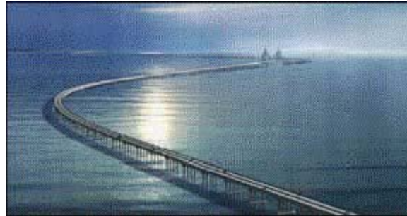
The Donghai Bridge
