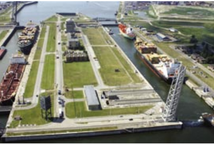
▲ To help ensure safe operation of the locks, the Zandvliet and Berendrecht lock areas were fully fenced off.
