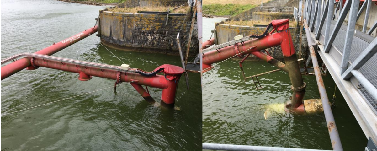
Figure 3.5. The beam construction holding the Tocado T1 tidal turbine in sluice 2 of Den Oever that was used to serve as a base for developing a robust housing construction to perform DIDSON measurements here.
