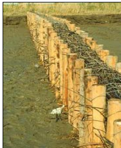
Fig. 10: Pier protection of tidal area.
