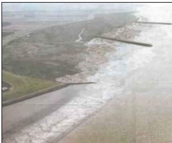
Fig. 9: Protection of eroding salt marsh near Waarde.
