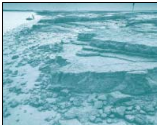
Fig. 6: Local erosion in intertidal area.
