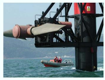
installed and commissioned 1km off Foreland Point, near Devon, UK, at a depth of 30 m. The device has a rotor of 15 m of diameter and it can generate a maximum of 300kW in a 2.7m/s current. A key patented feature of the technology is that the rotor and drive train can be raised completely above the surface for maintenance.
