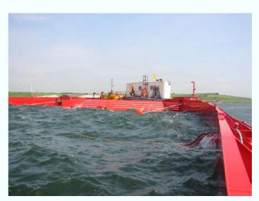
generation design. In May 2003, a  $57 \times 27$  m wide and 237 tonnes heavy 1:4,5 scaled prototype was installed and grid connected in Nissum Bredning. The prototype is fully equipped with hydro turbines and automatic control systems, and is instrumented in order to monitor power production, wave climate, mooring forces, stresses and device motion.
