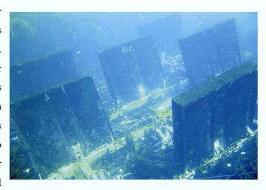
depth for installation is about 7-15 meters. As with all submerged wave energy conversion devices the device is characterized by low visual and acoustic impact.
