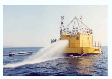
The device employs a patented, vertical axis rotor driving a synchronous generator. An important feature of the Kobold is that the direction of rotation of the rotor is independent of the current direction.
