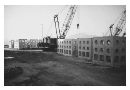
**Fig. 2.** Representative of efforts to incorporate biological design criteria into the physical structure of artificial reefs is the Box Reef, with open space in its upper level and confined space below (photograph courtesy of C. Kim).
