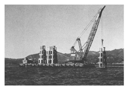
**Fig. 1.** Some of the largest artificial reefs, as used in commercial fishing in Japan (photograph courtesy of S. Otake).
