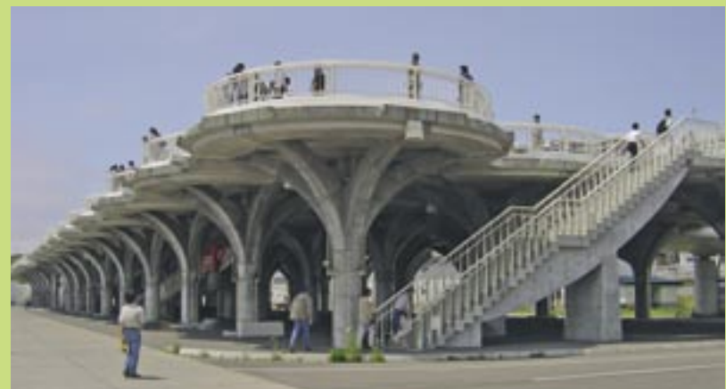
Evacuation platform at Aonae port
