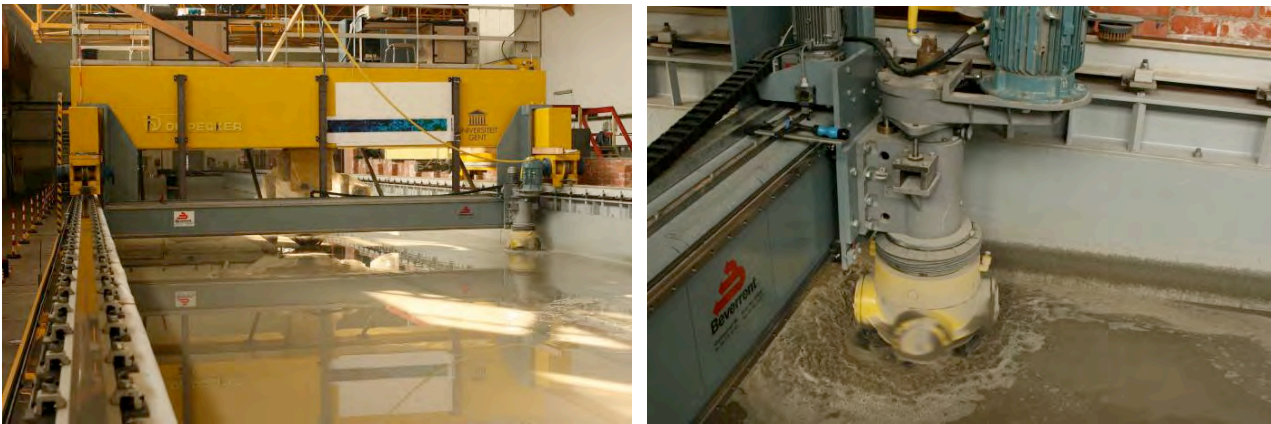
Fig. 17 - Flattening the bottom of the towing tank
