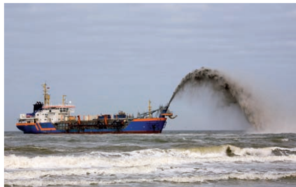
Figure 3.2. A dredger at work
