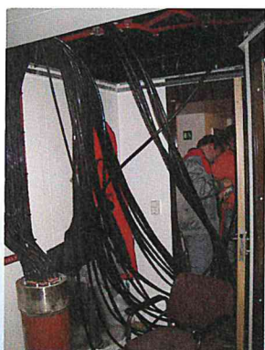
Almost 1.000 m of electrical cables had to be laid in the vessel
