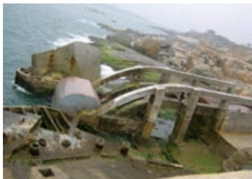
50 kW onshore oscillating buoy wave power device, energy buffer system, and desalination device
