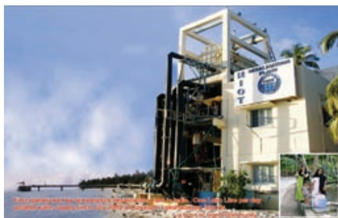
A view of the 100 m 3 /day Island Based Desalination Plant at Kavaratti, with an inset of Islanders getting the distributed water.
