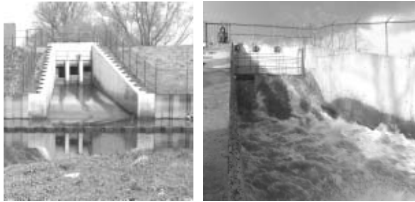
Photo 1.1 (left): Inlet culvert construction (as seen from within the pilot restoration site), consisting of three inlet culverts, each 1 m wide, with adjustable thresholds at different heights. Photo 1.2 (right): Close-up of the inlet culverts at spring tide flooding (as seen from within the pilot restoration site).
