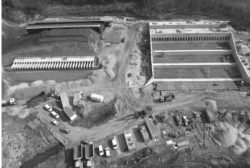
Photo 1.3: Aerial view of CRT construction along the Schelde. Photograph shows outlet (left) and inlet (right) construction which will allow implementation of CRT on several hundreds of hectares of lowered agricultural land.
