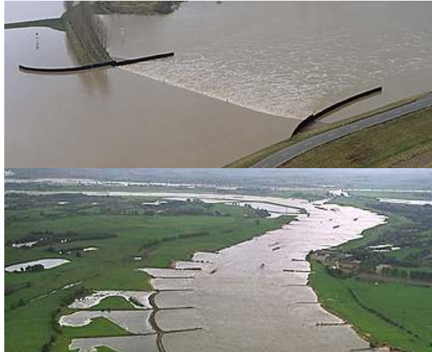
Figure 3.1: Weir flow (top) and groynes (down)
