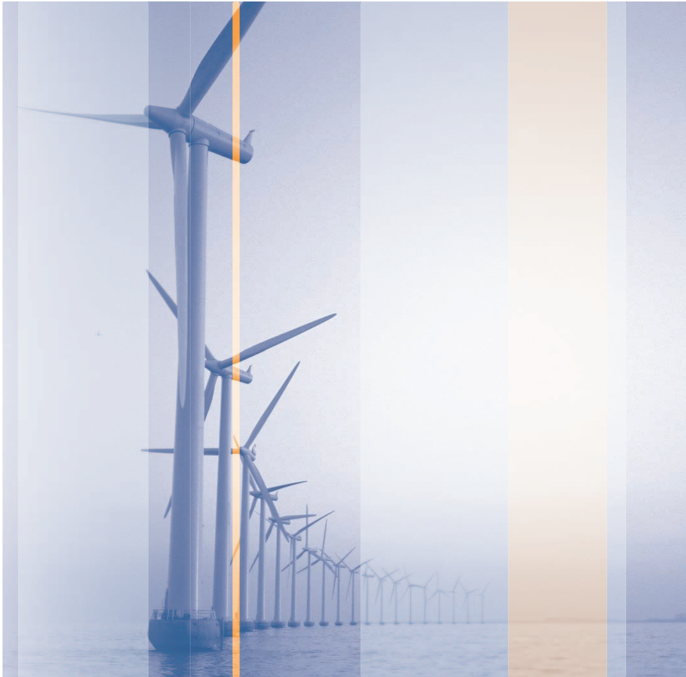
Middelgrunden wind farm, Denmark (© LM Glasfiber)
