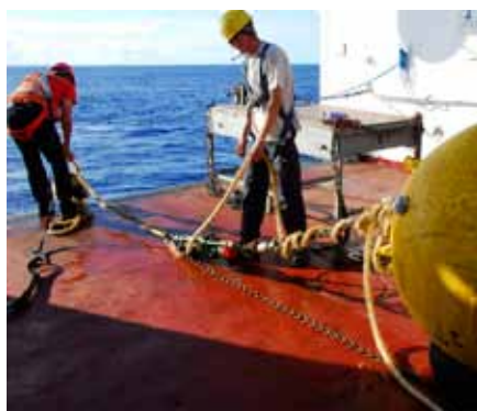
Top section of a RAPID mooring about to be deployed at 26N from RRS Discovery
