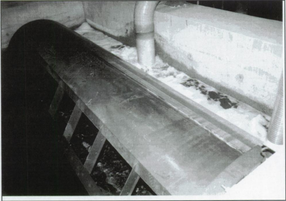
Photo 2.2.2 Cylinder shaped overflow weir
