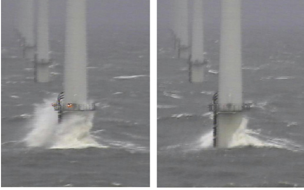
Fig. 1. Wave run-up on one of the towers of the Horns Rev wind mill farm; H_s=2.5 m, platform level=9 m above SWL, Elsam .
