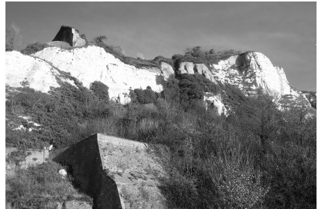
Fig. 2. East Cliff at Dover (Kent) showing the wall of Dover Castle truncated by cliff collapse. The Castle wall and cliff here are reported to have collapsed during the 1580 Dover Straits earthquake.
