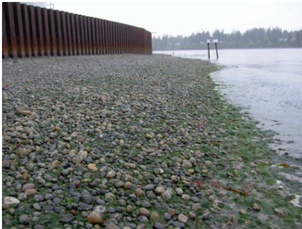
Figure 4 An intertidal bulkhead constructed of metal sheet pilings located on Puget Sound, Washington, USA. This bulkhead was built to retain contaminated sediments and reduce exchange with the sound.
