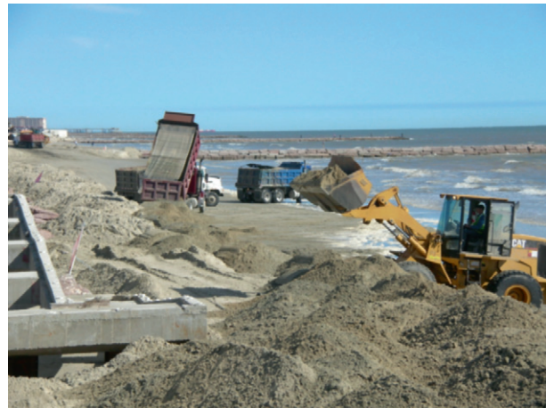
Figure 6 Beach-filling activities between rock groynes on the open coast of Galveston, Texas, USA in January 2009 following severe erosion and damage from Hurricane Ike.
