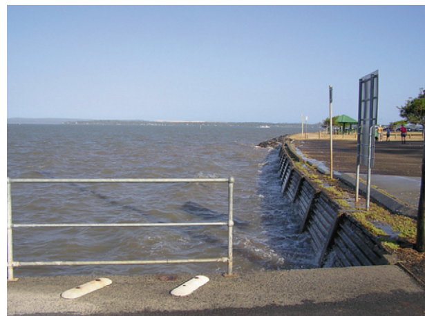
Figure 3 An example of a bulkhead built to protect coastal parkland at Redland Point, Queensland, Australia.
