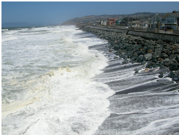
Figure 10 Beach loss seaward of coastal armoring that includes a seawall and revetment on exposed coast in Pacifica, California, USA. Note the lack of dry sand zones and lateral access for beachgoers.
