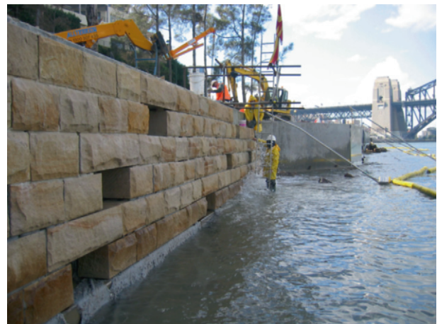
Figure 16 The construction of artificial rock pools in a new seawall being constructed in Sydney Harbour, Australia.
