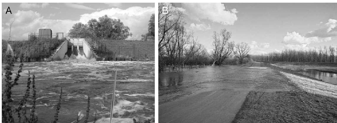
Fig. 2. Tidal energy dissipation operated through CRT system. A) Spring tide, inlet culvert. B) Storm tide, spillway; photograph, Droge voeten association (March 2008).
