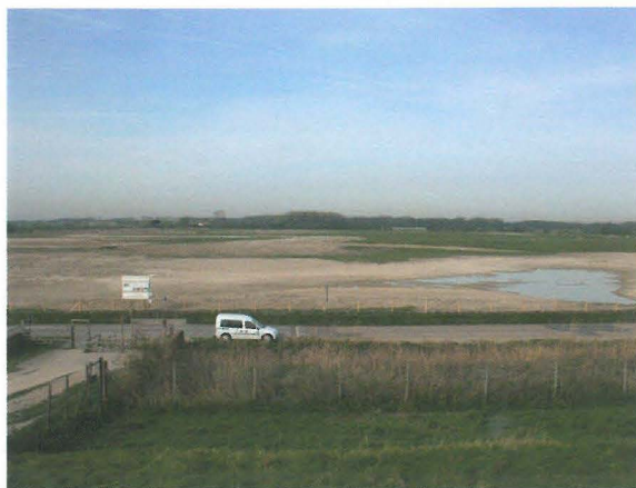
Figure 13. After the work (April 2010)
