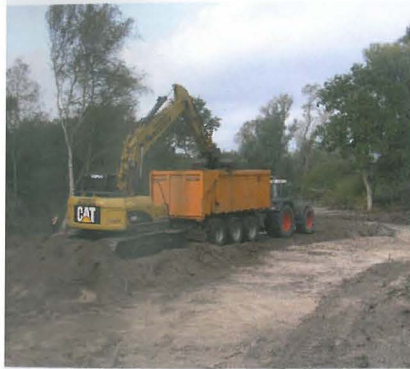
Figure 9. Cutting sods of grass in the western corner
