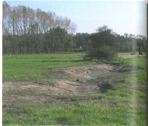
Figure 15. Show-jumping arena after the work (October 2007)
