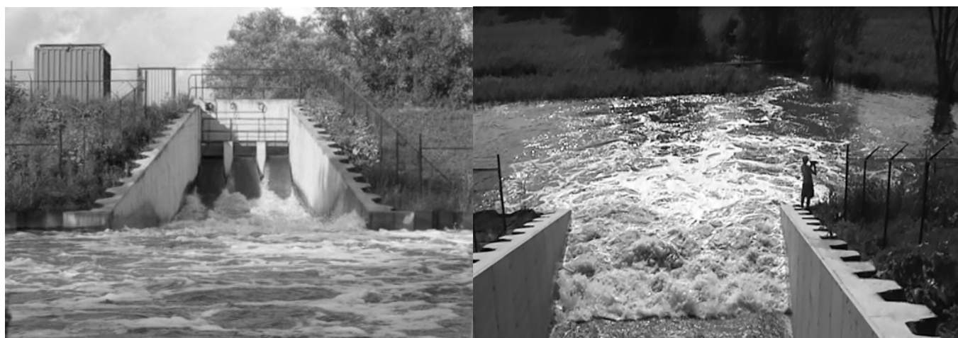
Figure 6. Energy dissipation and aeration of water flowing into FCA-CRT Lippenbroek (left: view from polder towards inlet sluice ; right: view from inlet sluice towards polder).
