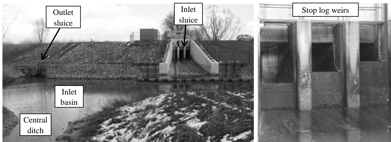
Figure 4. View from polder upon inlet sluice and outlet sluice of FCA-CRT Lippenbroek (left) and upon stop log weirs at downstream end of inlet sluice culverts (right)
