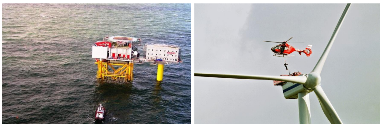
Figure 9: [Left] Offshore substation & living quarters at Horns Rev 2. [Right] Helicopter access for offshore maintenance
