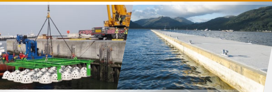
^ A floating breakwater was installed within 24 hours in Holy Loch, Scotland Picture: Intermarine Limited
