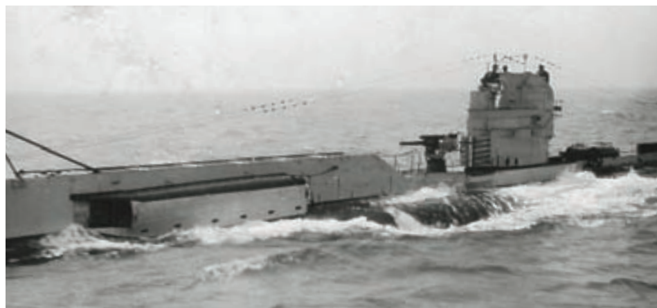
■ A UC-II type submarine at sea. This type of U-boat carried 18 mines in 6 internal chutes as well as a gun in front of the conning tower (Tomas Termote)
