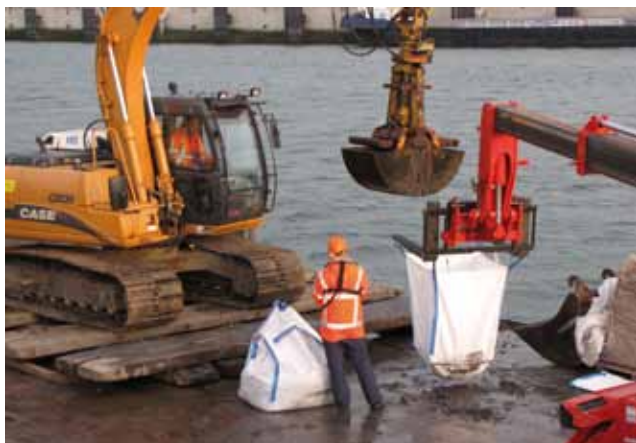
Fig. 2.21. The backhoe divided the soil from the container over two bulk bags, A and B.
