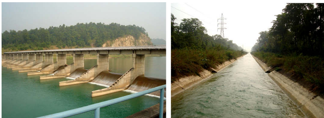
Fig. 2. The weir cum bridge across the Babai river (left) and the main canal (right).
