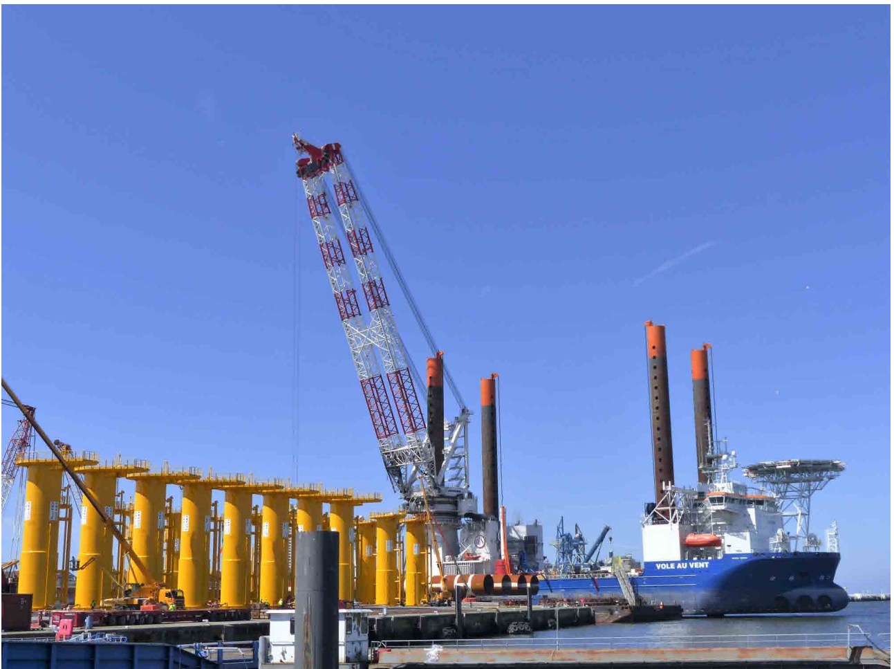
20 transition pieces (TPs) for Nobelwind on the Rebo terminal
