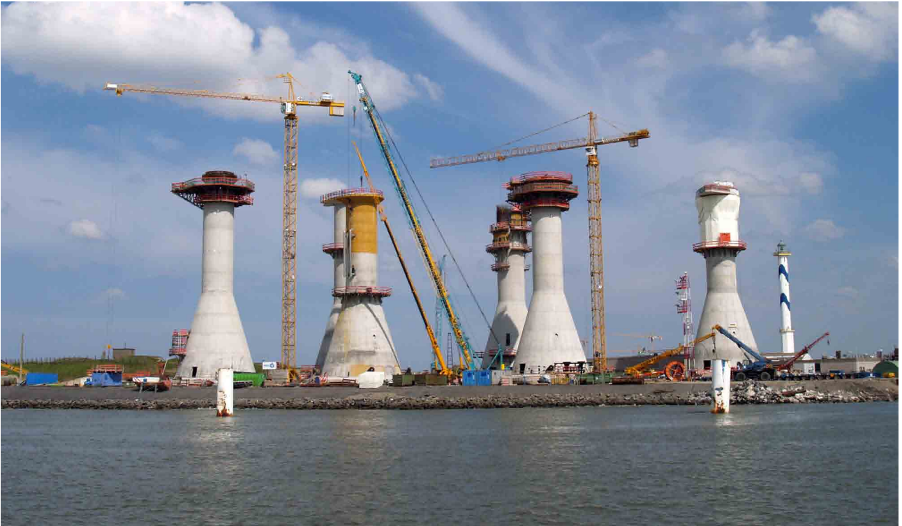
concrete foundations (GBF) for the first 6 wind mills in the C-Power park
