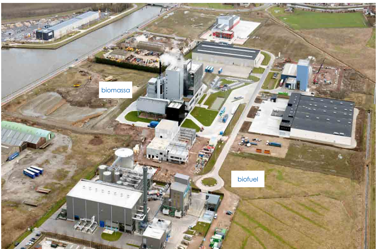
biomass & biofuel installation
