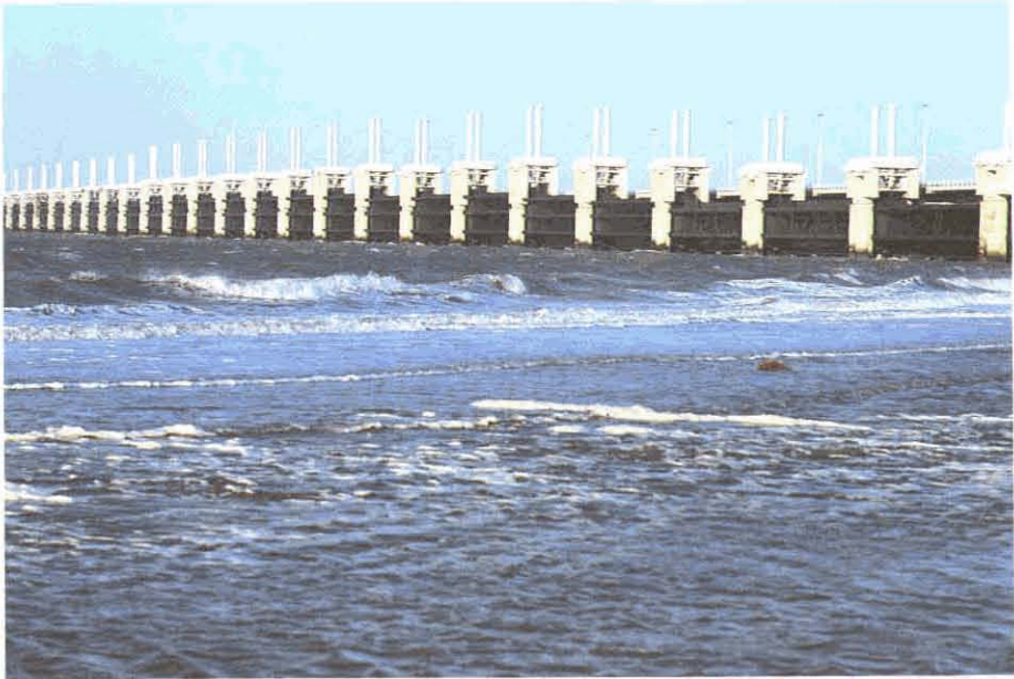
Storm surge barrier Eastern Scheldt
