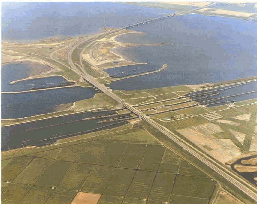
Volkerak dam and locks
