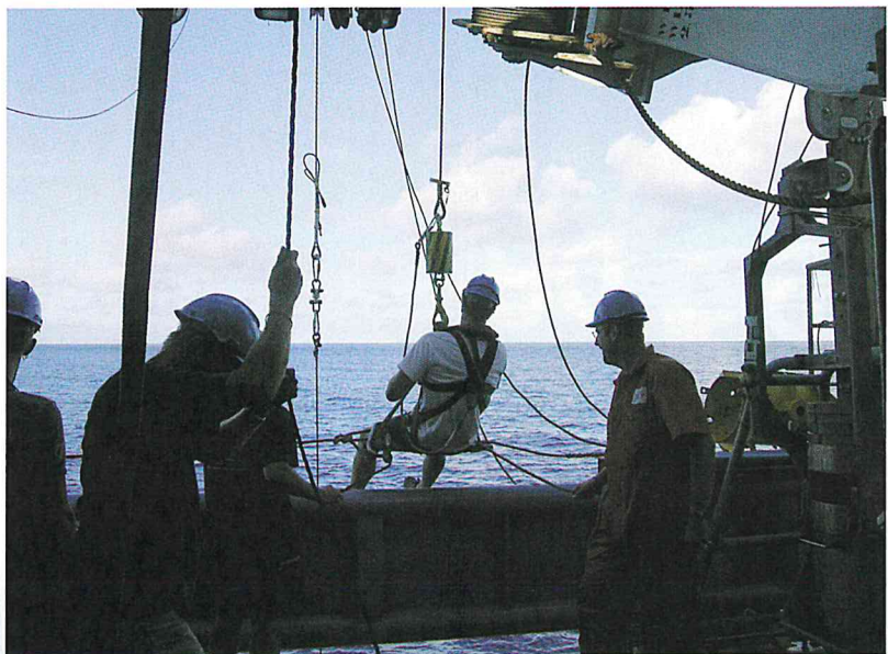
Repair work at A-frame of RV PELAGIA during MOUNDFORCE cruise
