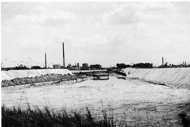
Fig. 71A — Sea-Scheldt dike. Slurry wall ditch.
