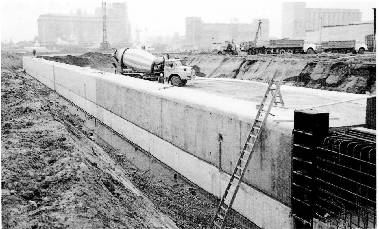
Fig. 56 — Quay wall section after being concreted.
