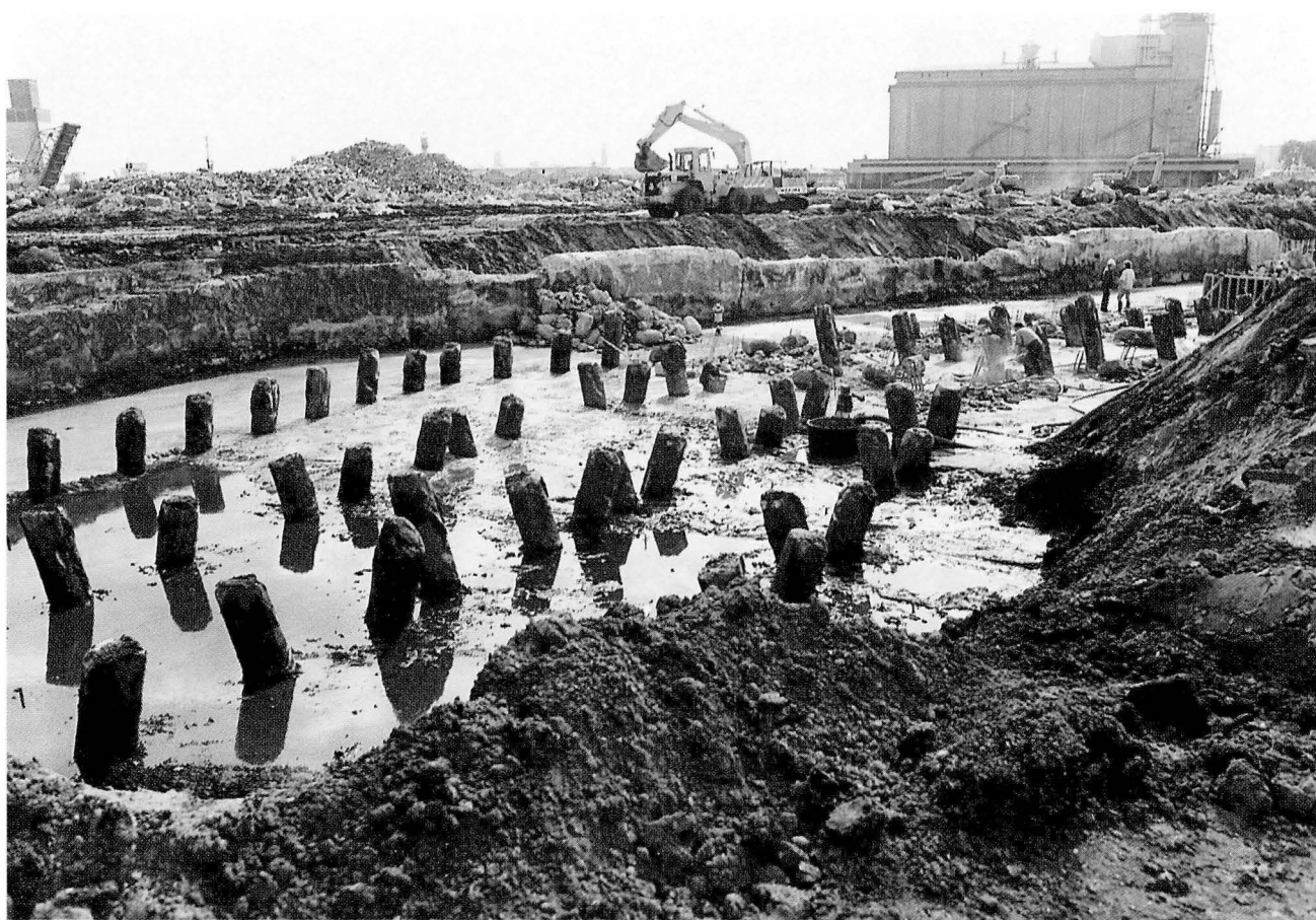
Fig. 51 — Pile heads after the excavation.
