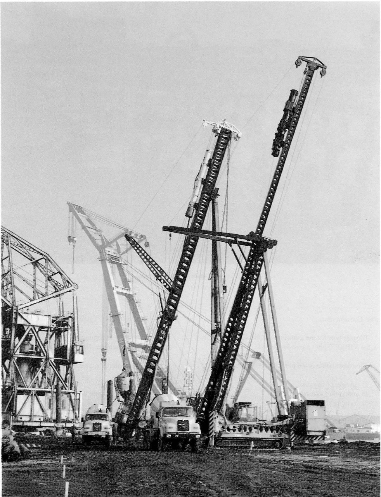
Fig. 50 — Construction of the vibrex-pile. Pile driving equipment. Background: derrick "Brabo" — Port Authority.
