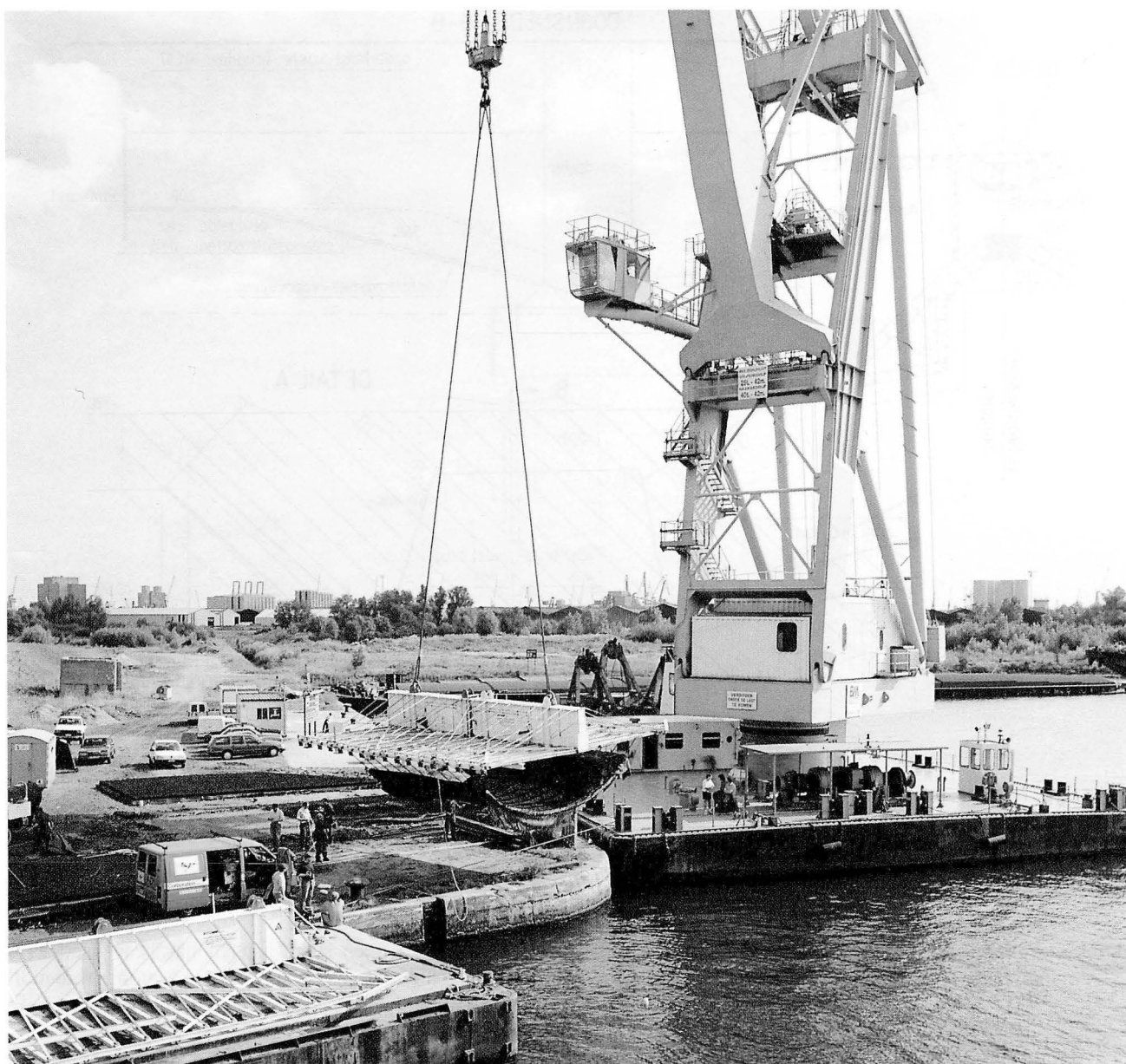
Fig. 73 — Prefabrication and laying of the stone asphalt mats under water.
