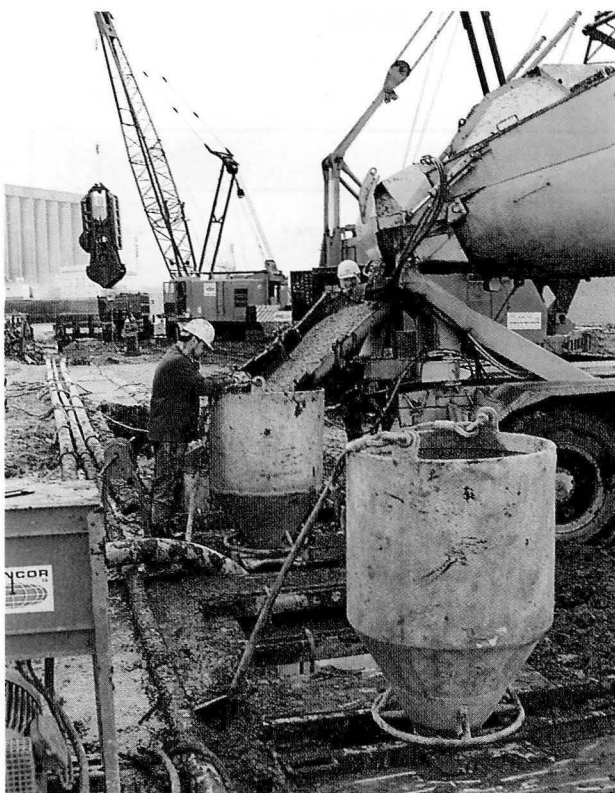
Fig. 40 — Slurry wall construction — panel concreting. Background: excavation of panel.
