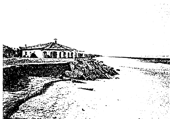
Fig. 2. Erosion problems near Punta Candor. The Quaternary cliff is eroded and summer houses are protected by a rip-rap revetment.
