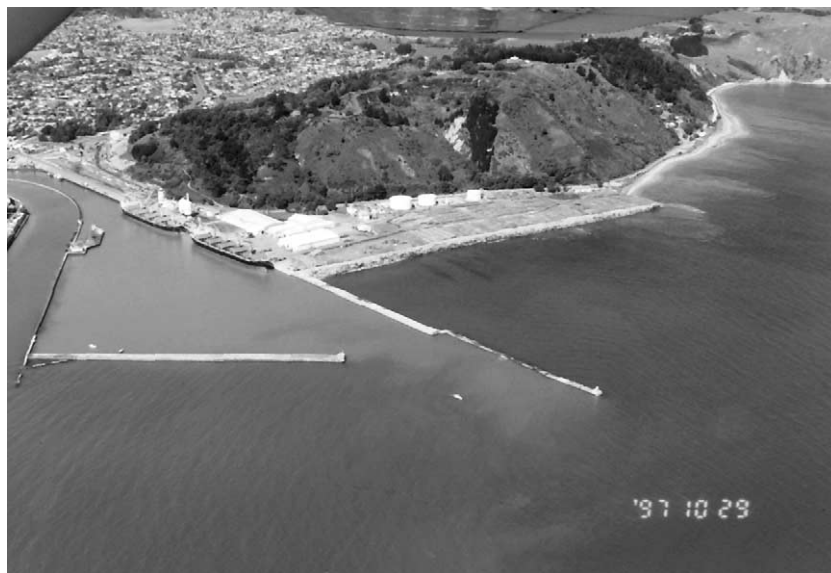
Fig. 3. Port outlay and present area of log storage. For redesign the reclamation is planned to extend along the shore platform, and the right breakwater will need to be removed.
