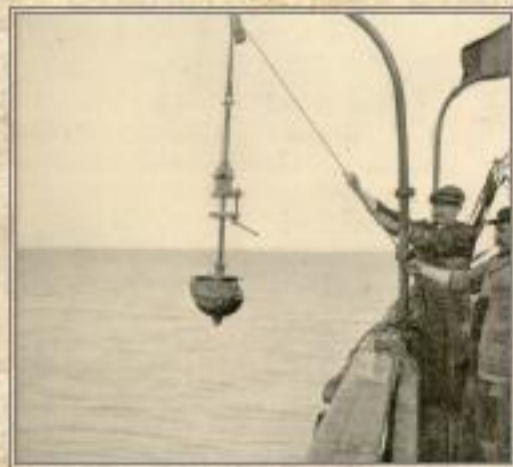
Figure 1 : The "ground-collector" filled with mud.
