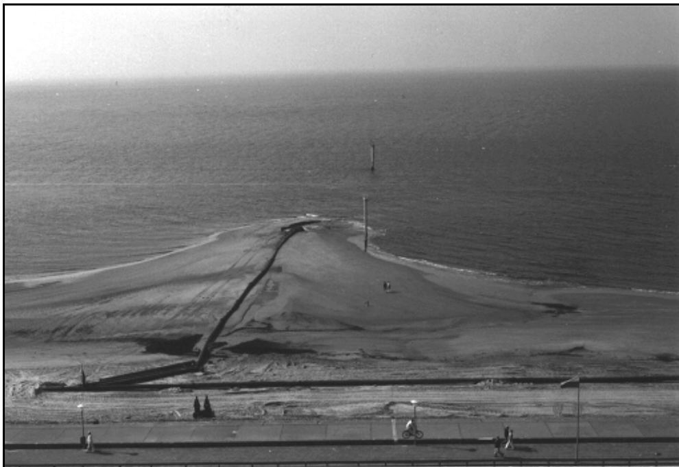
Figure 2. Execution of the shoreface nourishment by pumping humps of sand from the shore
