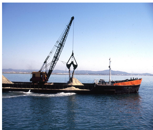
Figure 5.2. Channel dredging in coastal systems. Photo: R. Santos.
