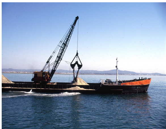
Figure 11.2. Dredging and sand reclamation from shallow coastal areas with seagrass beds has major detrimental impacts due to direct destruction of the beds and due to resuspension of sediments and reduction of the light conditions for plant growth. Photo: Rui Santos
