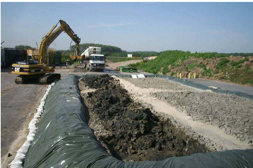
Figure 2.9: Lagooning fields during tilling with the excavator.
