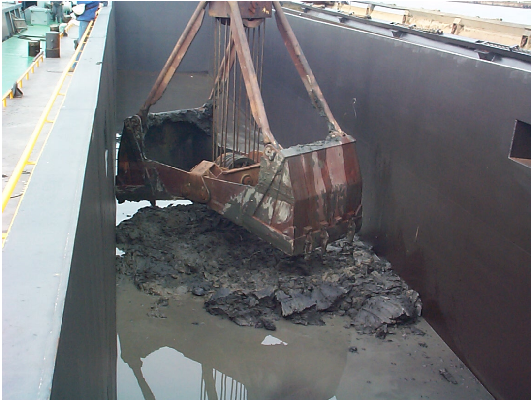
Figure 1.2: Transport of the sediments in a barge.
