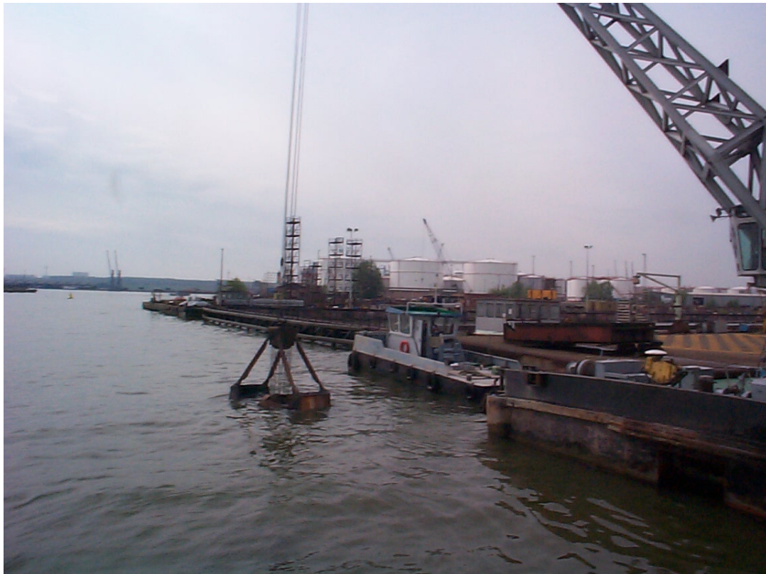
Figure 1.1: Dredging of sediment at location 1.5.
