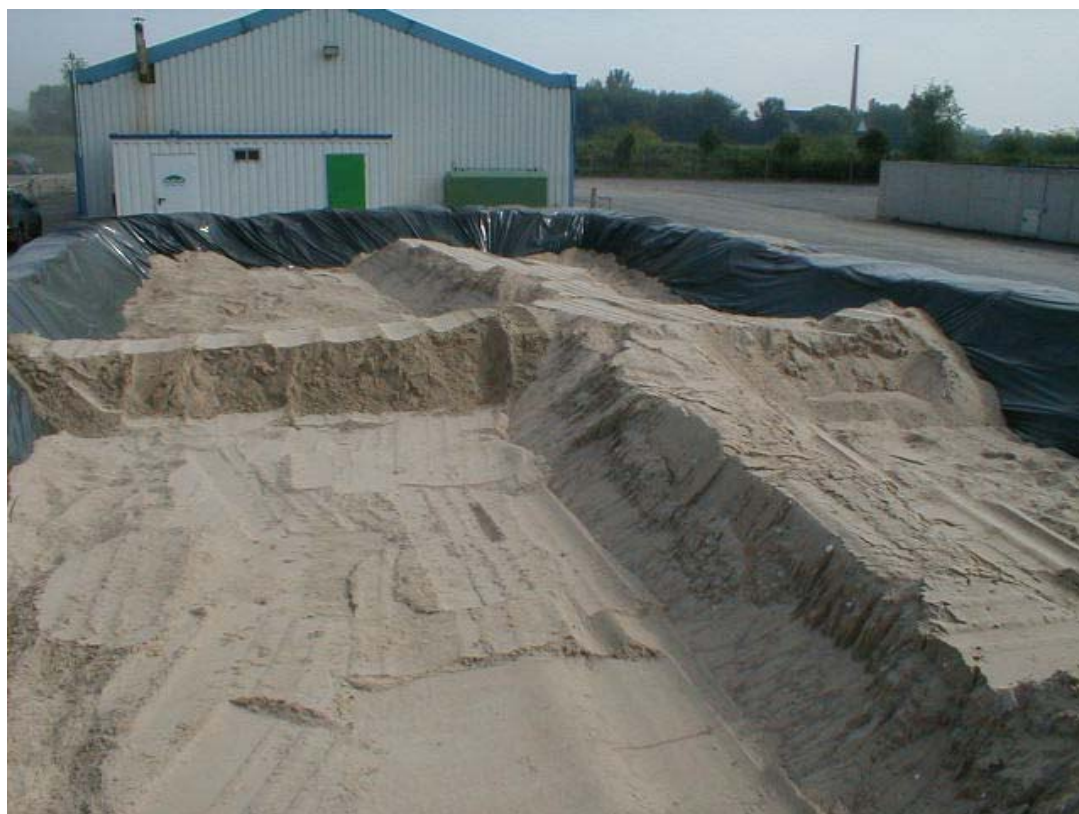
Figure 2.6: installation of the lagooning fields: drainage layers and separation dykes.
