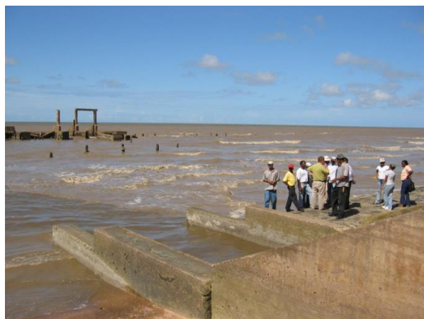
Coastal erosion in British Guyana – collapsing hard structure which should protect the hinterland.
