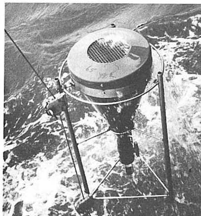
The funnel-shaped "Kiel-type" sediment trap was used in a free-floating manner during REFLEX.
