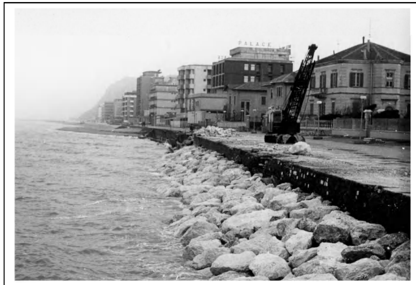
Plate 8.2 Rebuilding of the coastal road in Pesaro after sea-storm of the end of December 1978 (by Franco Marabini)
