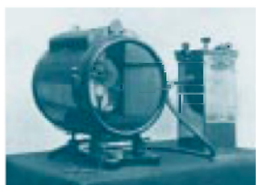
A blinker light was used to send Morse code messages at night.
