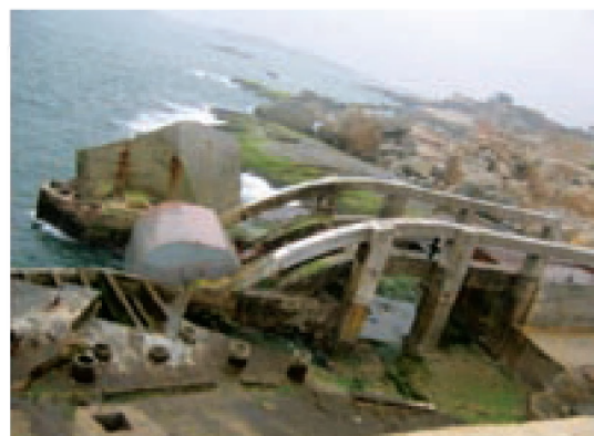
50 kW onshore oscillating buoy wave power device
