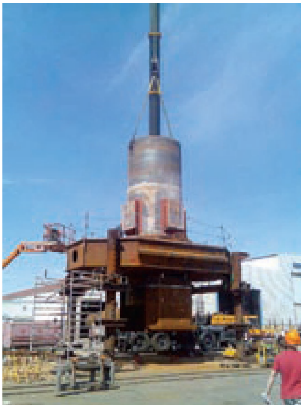
MCT SeaGen device – Pile and Collar
