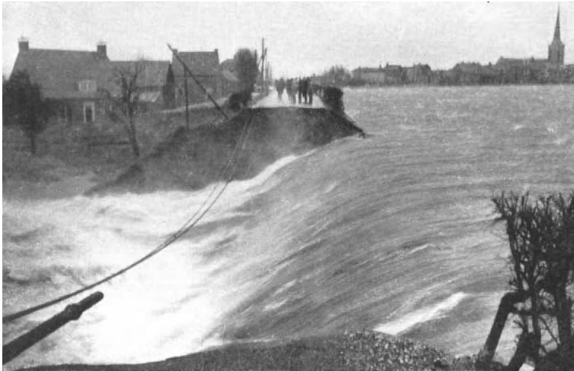
Figure 8. Breach at Ouderkerk aan de IJssel, upstream along the tidal reach of the river Hollandse IJssel, at the time of tidal low water (from Van Veen 1962 ).
