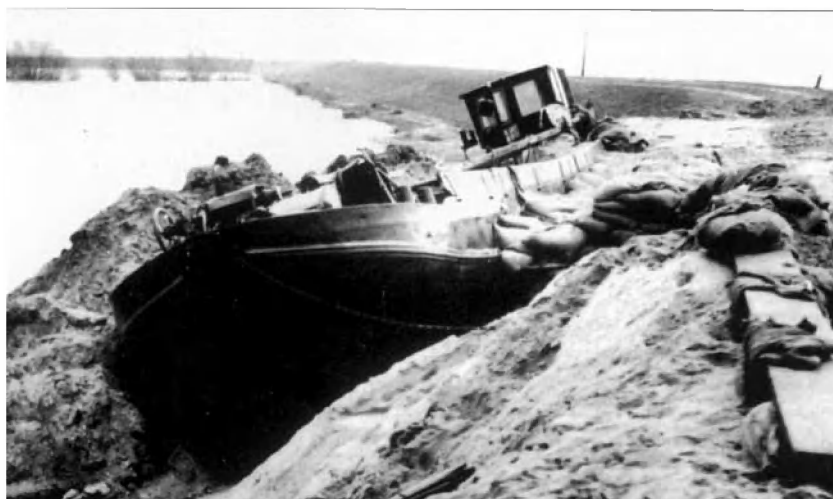
Figure 9. The ship that closed the dyke breach and saved the central parts of Holland from flooding (from Slager 1992 ; photo: C. van Gennip).
