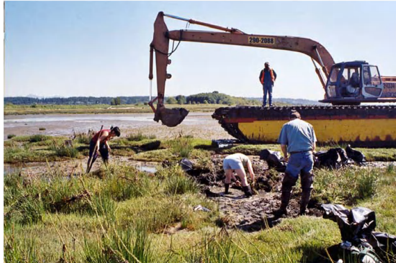
Figure 6 Swamp Excavator (photo by Pat Lim).
