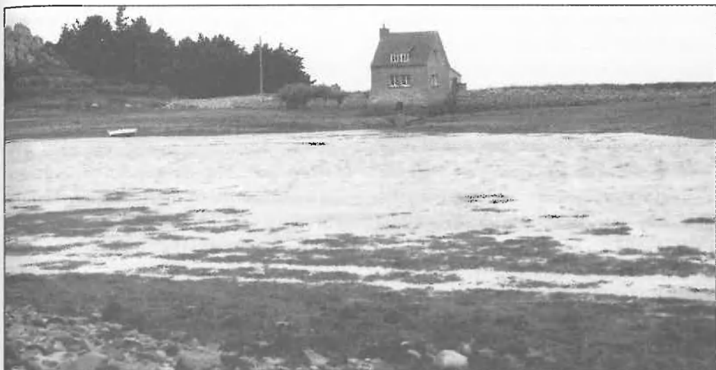
Fig. 7. The inter-island Buguelès Mill at Penvénan (Côtes d'Armor). This unique mill is built on a dyke between the Île Baëlenec and the Île des Oies. The funnel effect between the two small islands concentrates tidal energy and dispenses with the need for a mill pond. The mill building has become a private residence (Photo Loïc Ménanteau, 11/08/1993).
