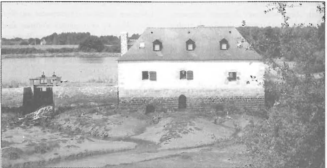
Fig. 6. The 17th century Mériadec Mill in Baden (Gulf of Morbihan, France) with dyke and two sluice gates with trap door. The mill stopped working in 1965. The 12.8 hectare pond, here seen at low tide, was used for aquaculture (Photo Loïc Ménanteau, 21/08/1993).
