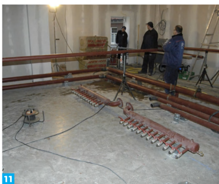
9. The diesel generator that will provide an emergency power supply arrives. | 10. Pipework of the thermal storage system on the roof. | 11. Interior pipework of thermal storage system. | 12. The final tile is laid.
